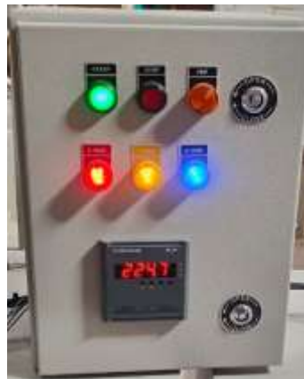
Fig 10: ON Function of DOL Starter
